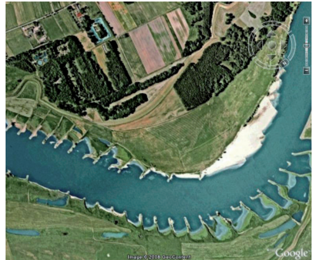
Figure II.4.35. A groyne system on the river Elbe, at km 477. The gravel bank on the inside does not obstruct navigation.
