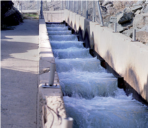
Figure II.4.23. Example of a pool and weir fish ladder, allowing fish to bypass the dam and reach the higher water level through a series of low-head weirs
