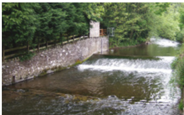
Figure I.7.13. River Grwyne at Millbrook: South Wales. Single crest crump weir
