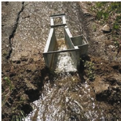
Figure I.8.2. Modified 3-inch Parshall flume in use
