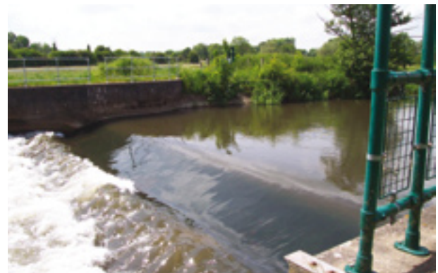
Figure I.7.12. River Kennet at Theale. South East England. Single crest crump weir.
