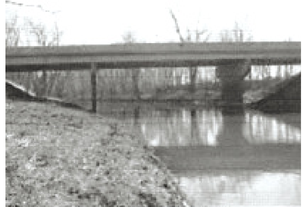
View, looking upstream
