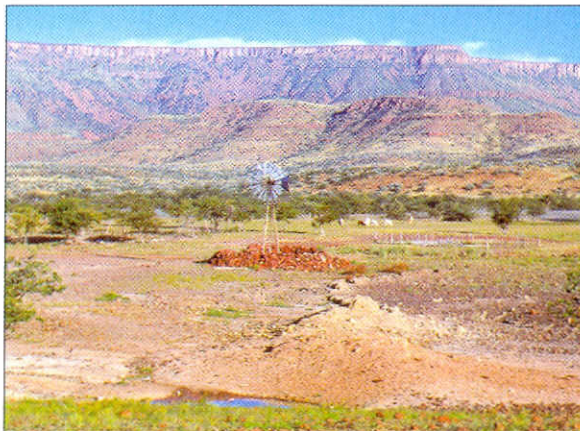
A rock wall can be used to protect borehole installations from thirsty elephants.
