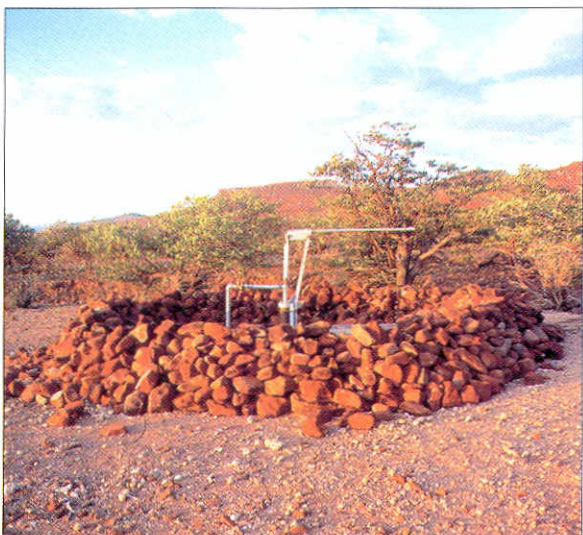
Water development in the absence of land use planning is a common theme in the western catchments. This borehole, installed to provide water for livestock during the 1993 drought relief programme, was sited in the Uniab catchment - a key area for tourism and conservation. The rock wall around the pump protects it from elephant which are common in the area.
