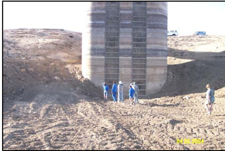
Photo 7.3.1: Omdel Dam after the removal of the silt around the abstraction tower.
