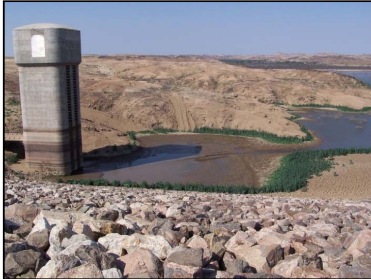
Photo 7.3.2: Dead storage water of Omdel Dam is canalled to the abstraction tower.
